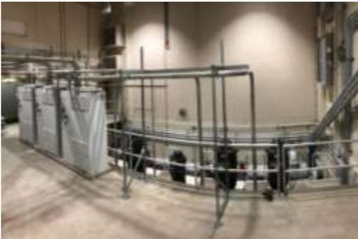
Work included replacing old pumps with higher capacity pumps and providing modern control technology.
